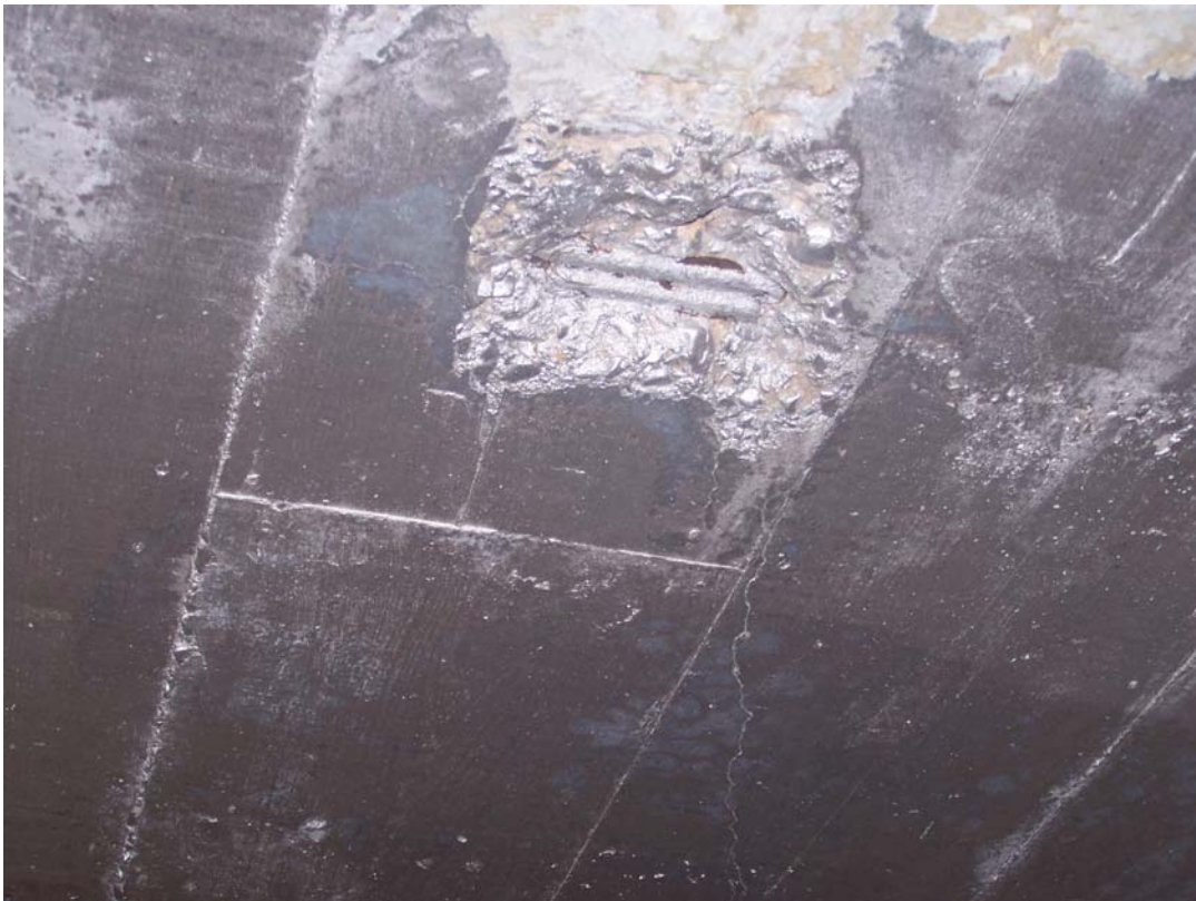
Photo 172 Painted spall in ceiling of room 6.
