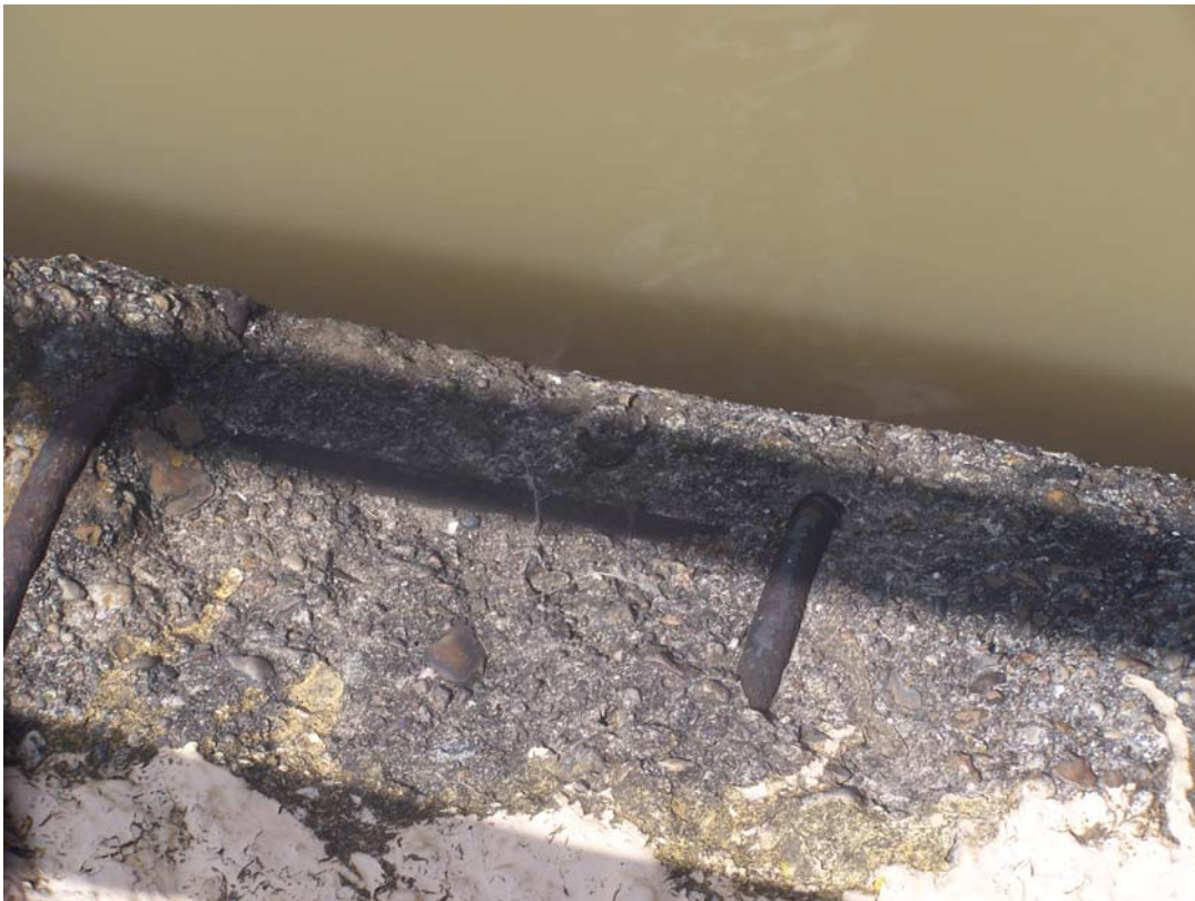
Photo 147 Spalls in east lock chamber wall. (Typical).
