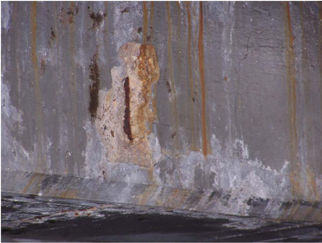
Photo 51 Popout in beam over gate 1 hinge.
