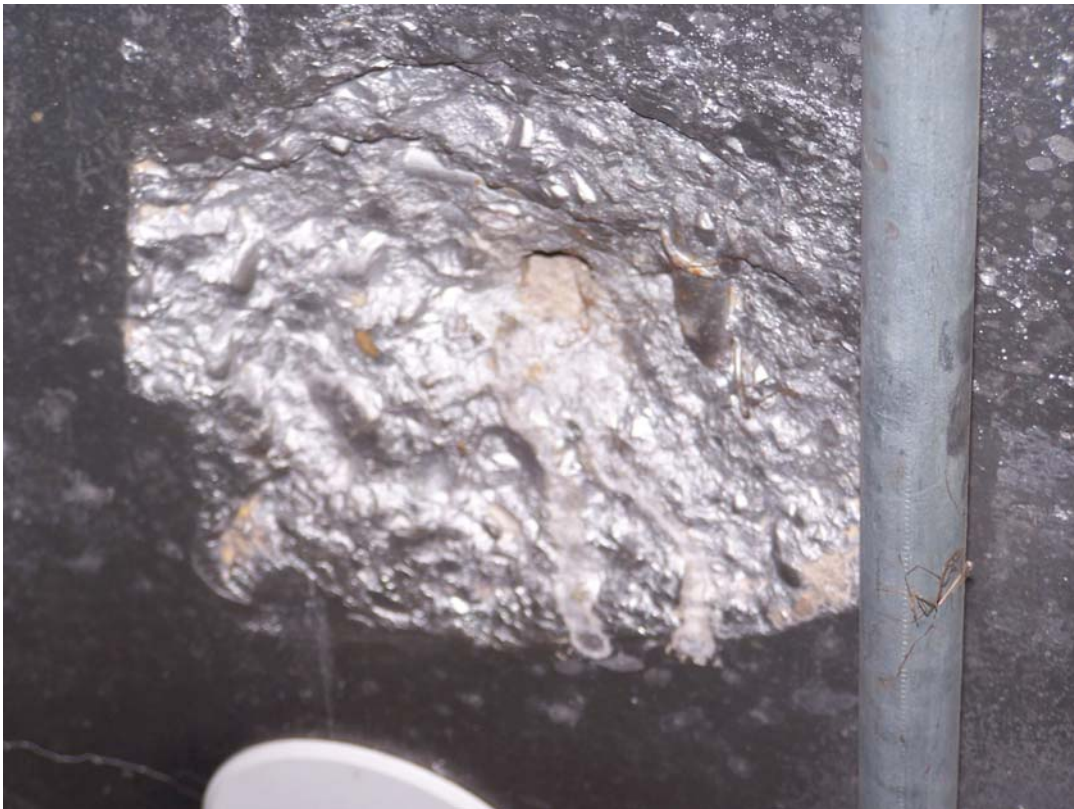
Photo 52 Popout in beam over gate 1 machinery.
