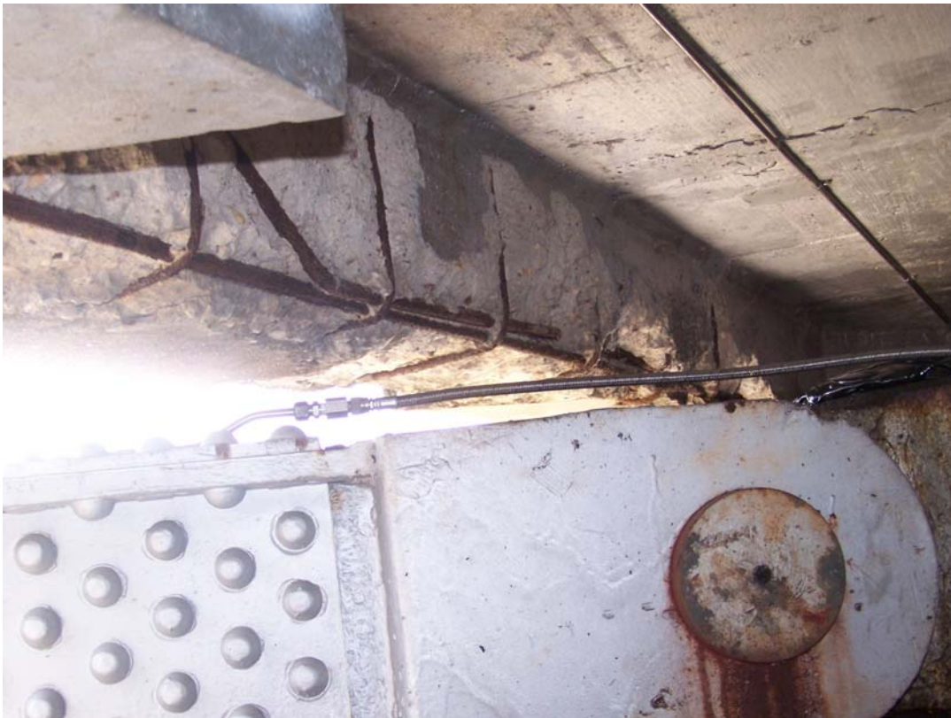
Photo 128 Deteriorated beam over opening for Gate 5.
