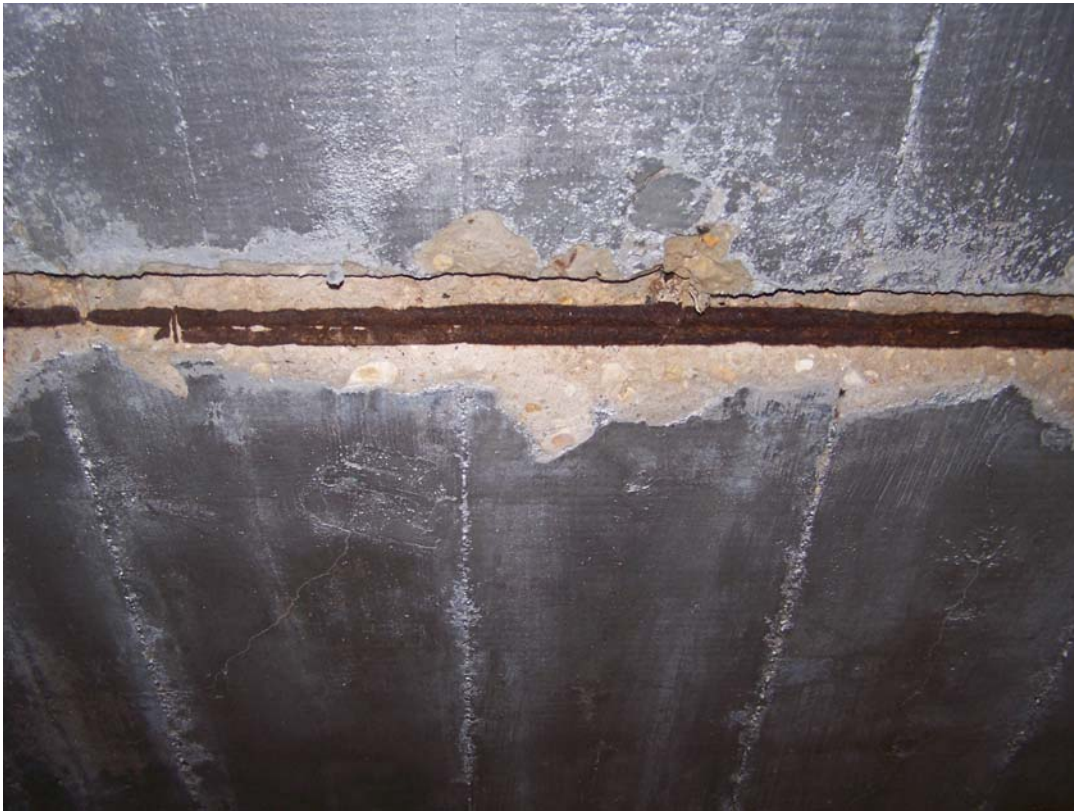
Photo 119 Spalls in ceiling near gate 5.
