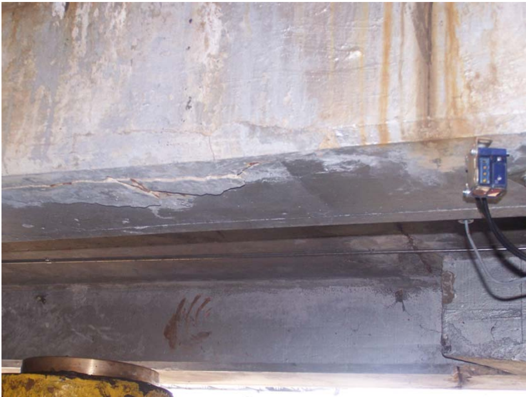
Photo 160 Crack in beam in Room 2.
