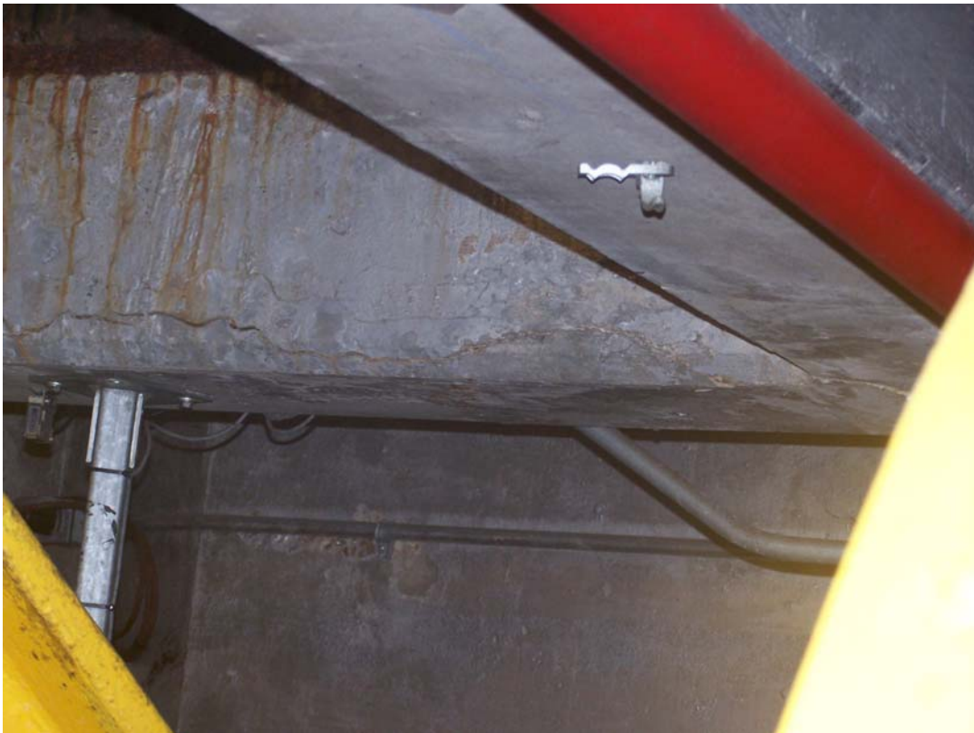
Photo 162 Crack in beam over Gate 4.
