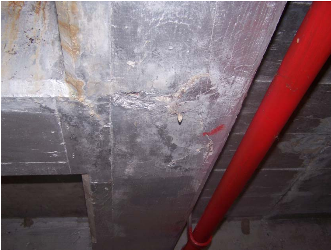
Photo 176 Cracks in beams by hinge in Room 6.
