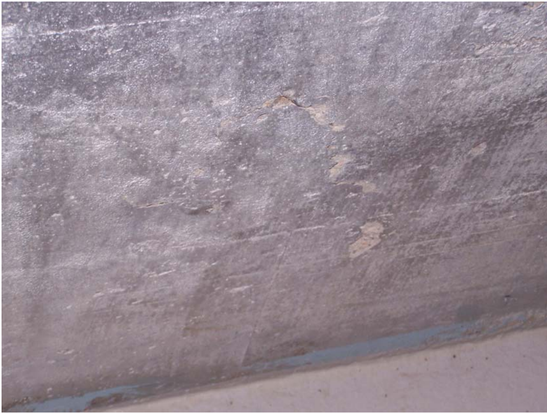
Photo 77 12" x 7" delamination in west tunnel wall.
