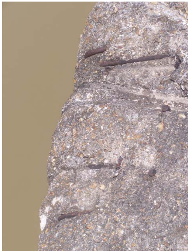
Photo 146 Spalls in north gatebay.
